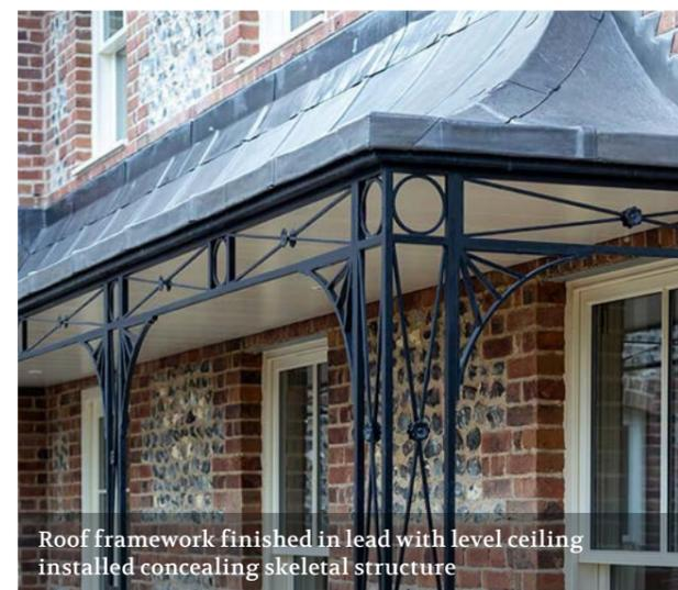
Roof framework finished in lead with level ceiling installed concealing skeletal structure
