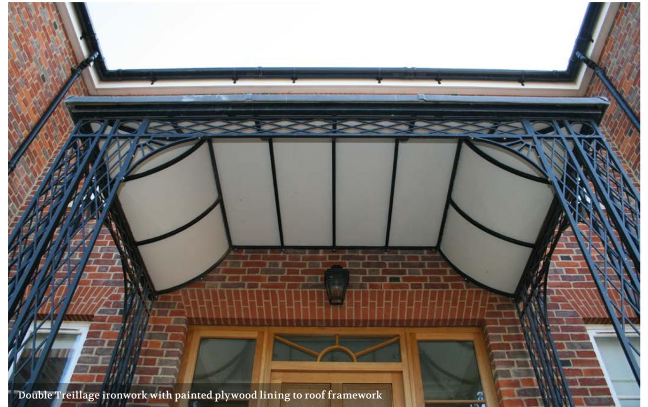
Double Treillage ironwork with painted plywood lining to roof framework
