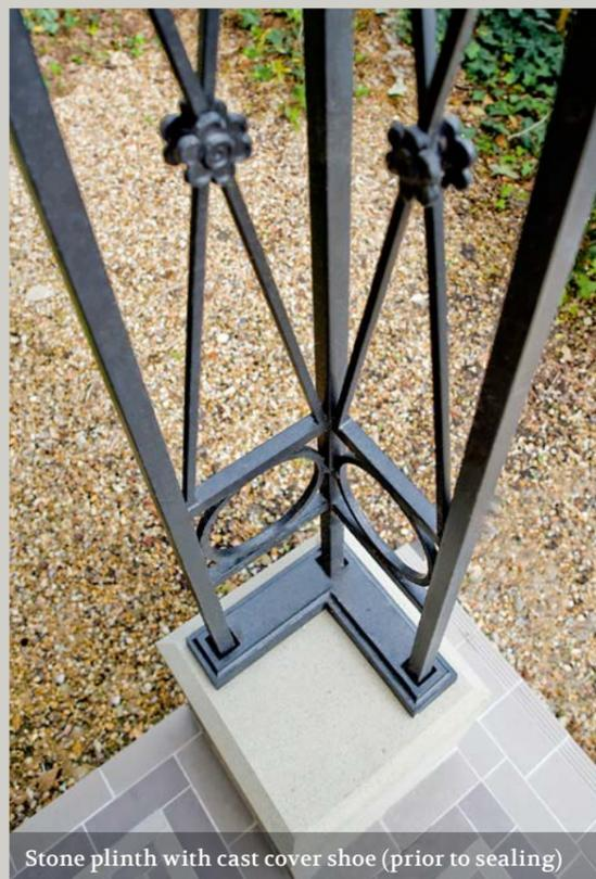
Stone plinth with cast cover shoe (prior to sealing)
